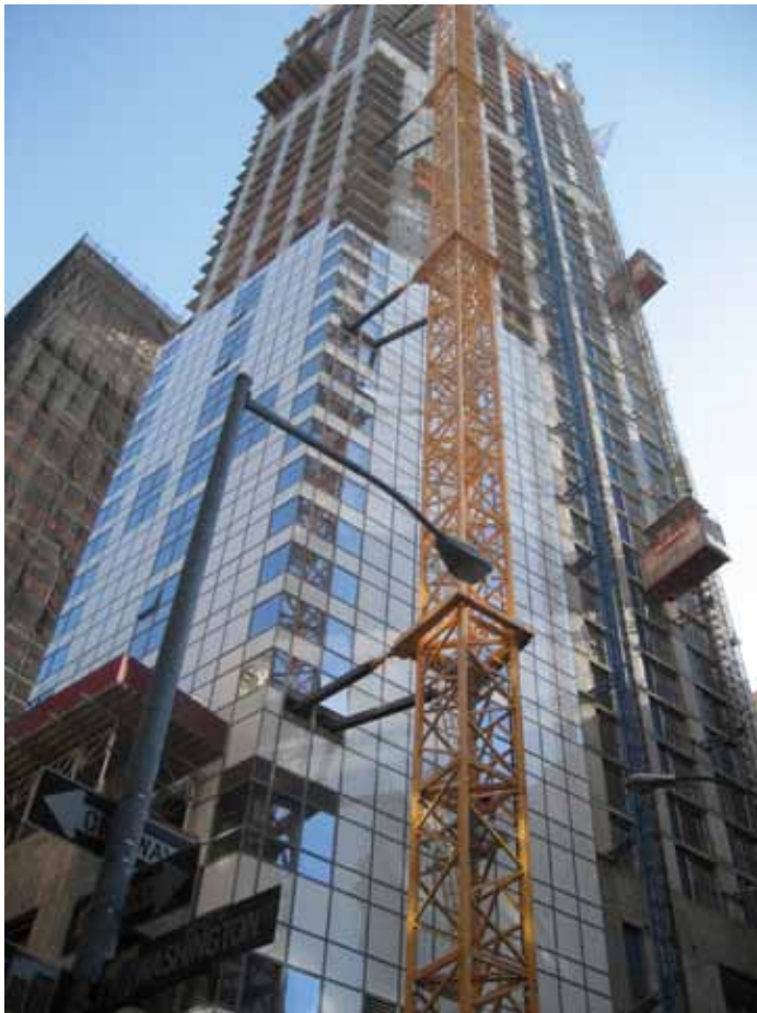
Figure 2: Construction of W New York Downtown Hotel and Residence.
